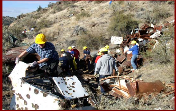
Willow Creek Dump Site Clean-Up
