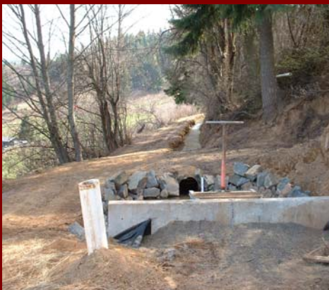
Current terminus of the Central Canal Upgrade pipeline (constructed in 2004-2005).
