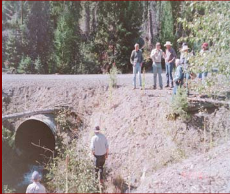
Forest Culvert Project
